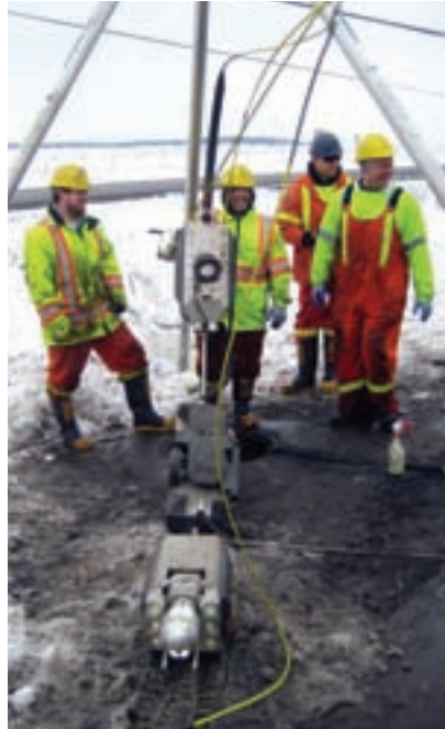
Crew ready to insert the robotic device into the water main
